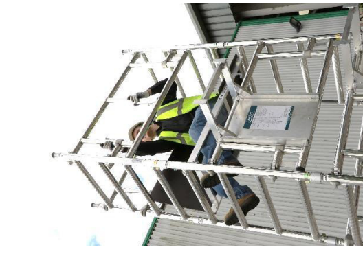
23. Retrieve a side guardrail frame from the front assembly bracket and locate it as shown.
