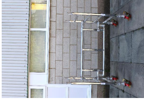
2. Fit a guardrail frame to the vertical member above the 3 rd rung with the hooks facing outwards.
