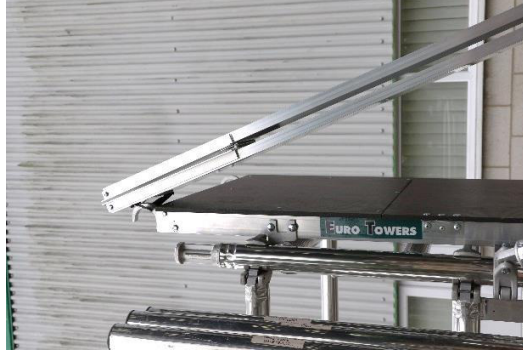
17. The toeboard can be located over the platform hook using the dedicated hanging strap.
