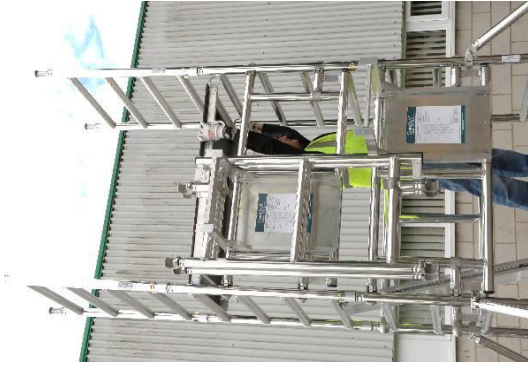
22. Repeat this process for the opposing side, ensuring that all interlock clips are engaged.
