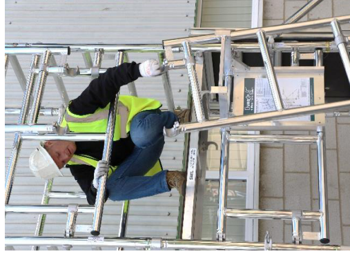
23. Retrieve 2 stowed side guardrail frames from the lower assembly bracket (front) pass them up to be relocated on the higher assembly bracket.
