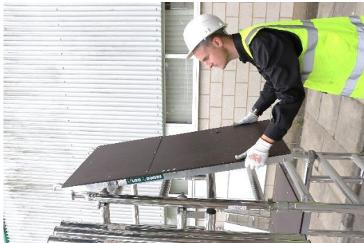
11. Remove toeboard and fit 2 assembly brackets in the position shown (side and front)
