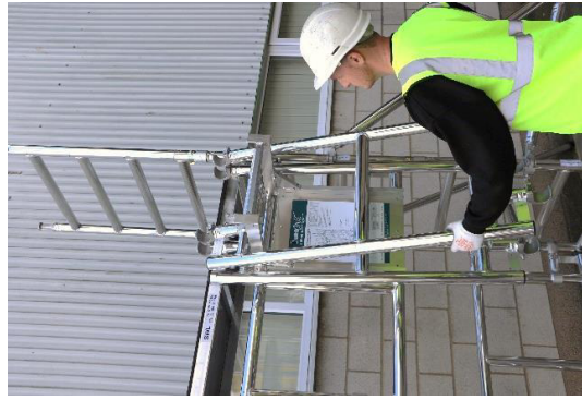
11. Stow the guardrail frames on the front assembly bracket.
