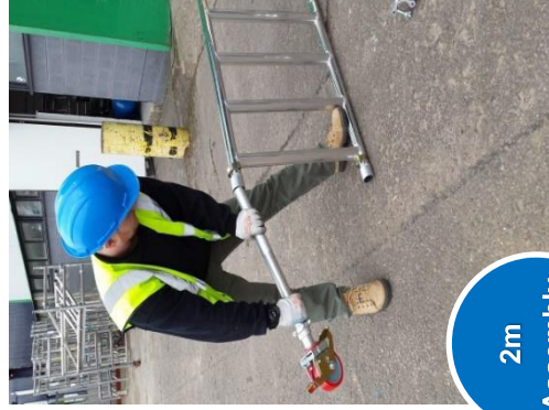
1. Insert legs and castors into a pair of frames.
