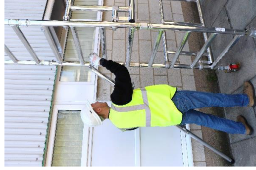
7. Fit 4 stabilizers, one on each upright of the tower.
