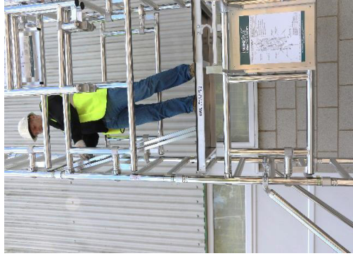
25. Temporarily locate the toeboard assembly on the platform to allow access to the additional platform that is stowed.
