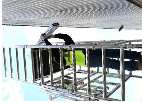
28. Relocate the toeboard assembly from the lower platform to the higher level, ensuring that it is positioned on the plain section of the platform as shown.
