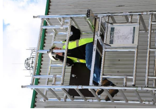
29. Fit 2 guardrail frames, with the top hook (facing outwards) set above the top rung of the frame.
