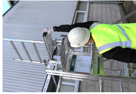
12. Relocate the toeboard assembly from the lower platform to the higher level, ensuring that it is positioned on the plain section of the platform as shown.
