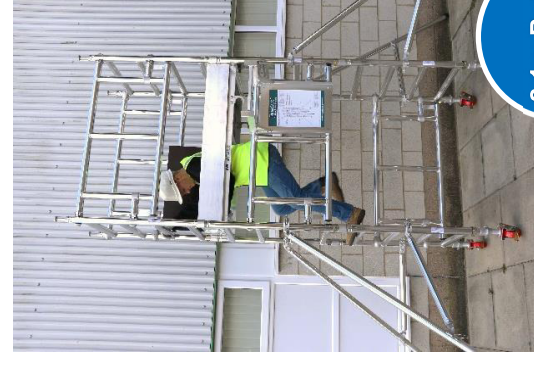
15. Access the platform using the trapdoor as shown and begin work.
