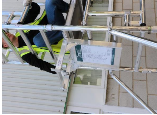
21. Relocate the "empty" assembly bracket from the side of the tower.
