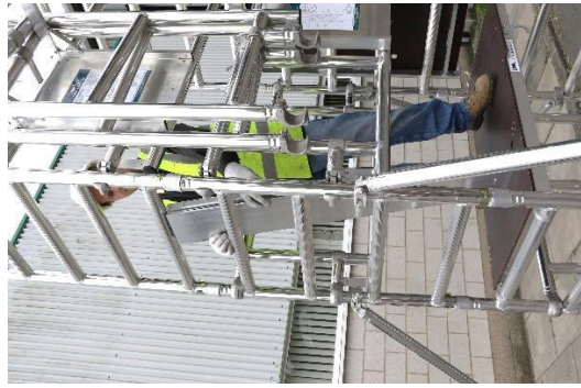
26. Temporarily locate the toeboard assembly on the platform to allow access to the additional platform that is stowed.
