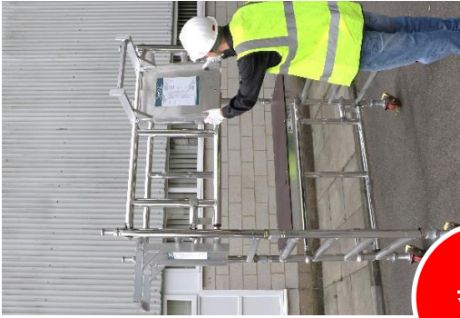
11. Remove toeboard and fit 2 assembly brackets in the position shown (side and front)
