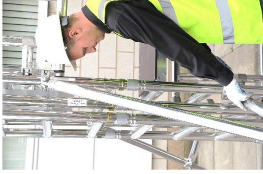
19. Fit 4 stabilizers, one on each upright of the tower.
