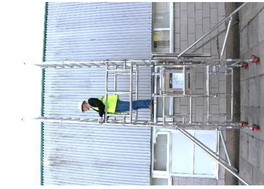
18. Repeat this process for the opposing side, ensuring that all interlock clips are engaged.
