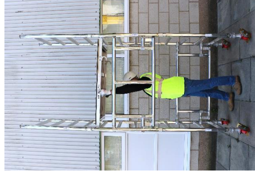
6. Fit the platform, 1 rung above the side frame location as shown.
