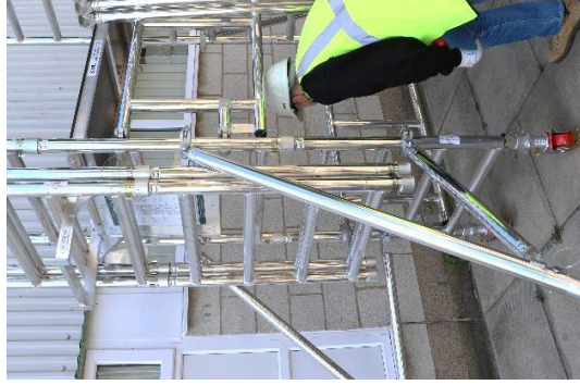
20. Access the platform by passing under the side frame and via the trapdoor platform.
