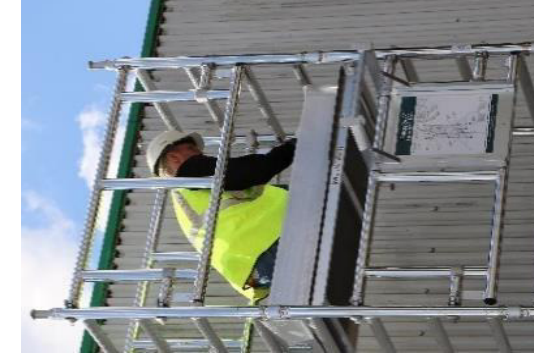
14. Fit toeboard by unfolding the set above the platform (please use labelling as a reference to ensure that the toeboard is the correct way up).
