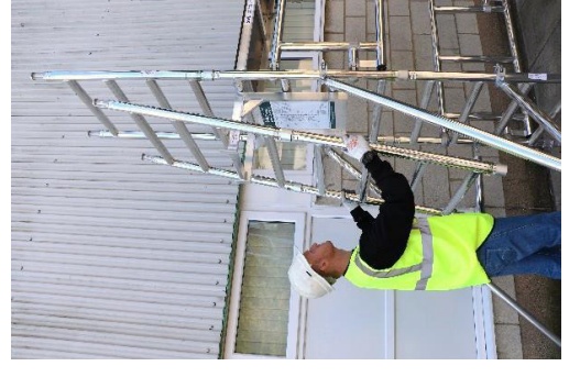
10. Stow the frames on the side assembly bracket
