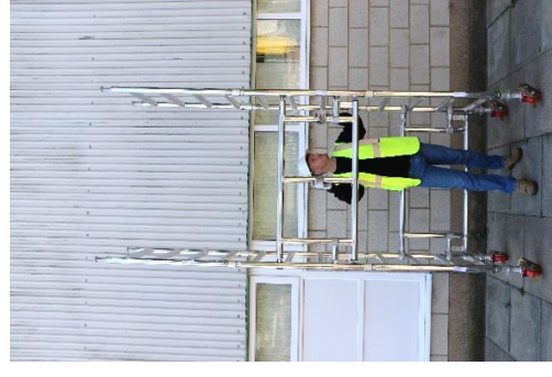
5. Fit 1 guardrail frame above the 7 th rung. Hooks facing outwards. (Refer to labelling to ensure that the frame is the correct way up)
