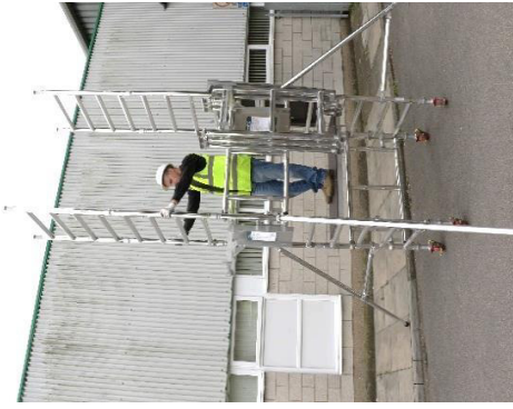
22. Repeat this process for the opposing side, ensuring that all interlock clips are engaged.
