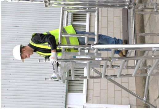
21. Retrieve a set of frames from the side assembly bracket and fit.
