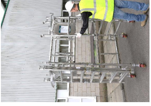
15. Stow 3 guardrail frames on the front assembly bracket.
