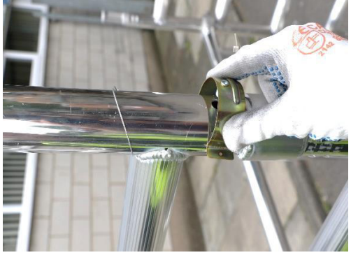
13. Engage interlock clips.
