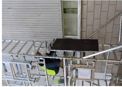
26. Remove the remaining platform from the lower section of the tower and pass up through the side frame.
