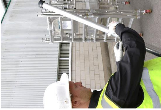
18. Before fitting stabilizers, release the pin to enable extension.
