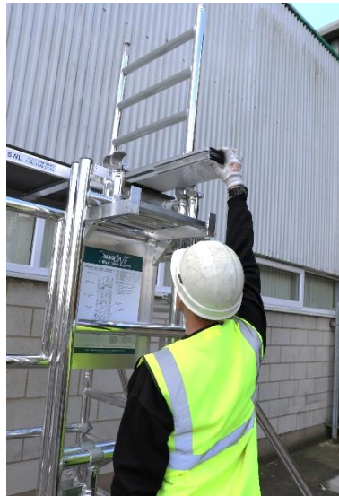
12. Relocate the toeboard assembly from the lower platform to the higher level, ensuring that it is positioned on the plain section of the platform as shown.
