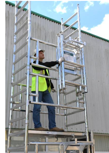
24. The frames are relocated as shown.
