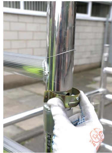
13. Engage interlock clips.
