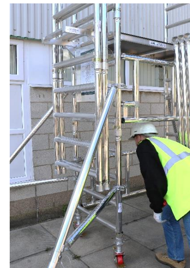
20. Access the platform by passing under the side frame and via the trapdoor platform.
