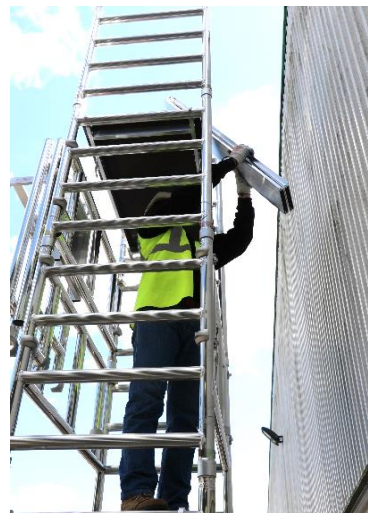
28. Relocate the toeboard assembly from the lower platform to the higher level, ensuring that it is positioned on the plain section of the platform as shown.
