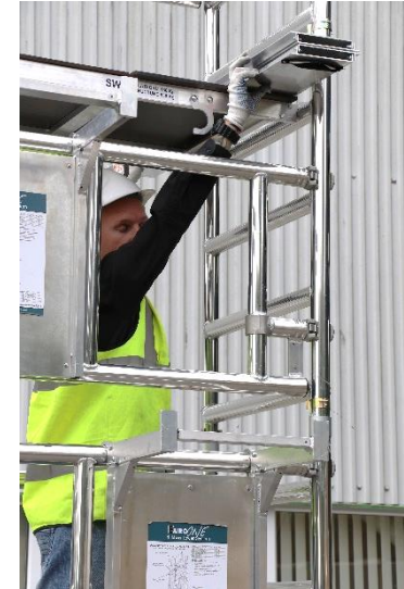
29. Relocate the toeboard assembly from the lower platform to the higher level, ensuring that it is positioned on the plain section of the platform as shown.
