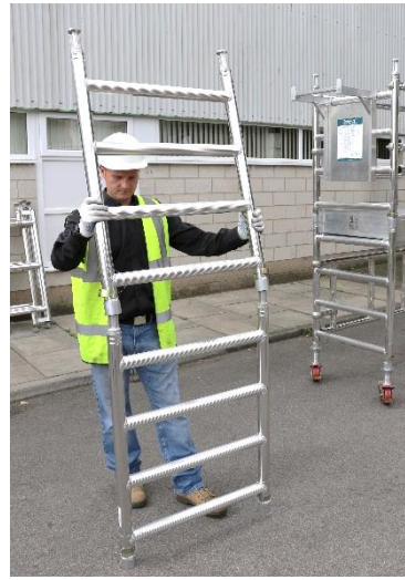
12. Assemble the frames in pairs as shown.
