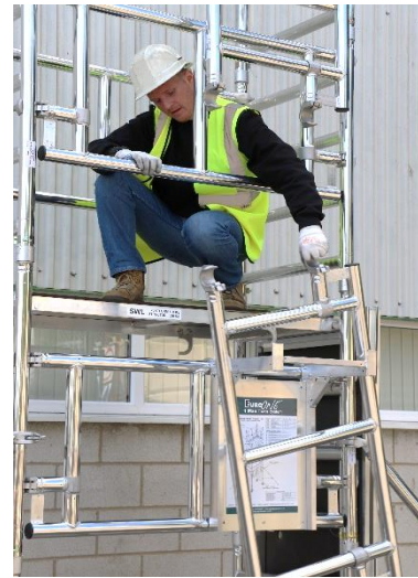
23. Retrieve 2 stowed side guardrail frames from the lower assembly bracket (front) pass them up to be relocated on the higher assembly bracket.
