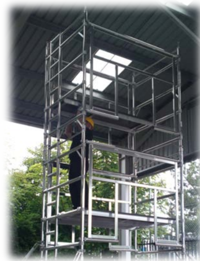
14. Remove the temporary trapdoor platform Position to the appropriate rung (Trapdoor facing the ladder section) 1 rung above the bottom section of the AGR frames.
