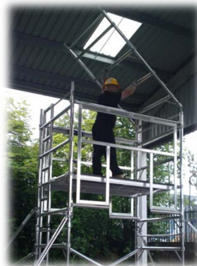
11. Add 4 rung frames, ensuring that the ladder is continuous.
