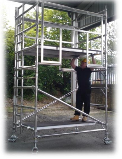
8. Position the trapdoor platform to the appropriate rung (Trapdoor facing the ladder section) 1 rung above the bottom section of the AGR frames.
