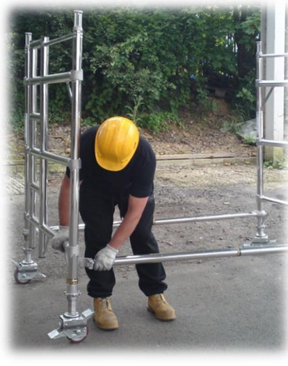
2. Klik in 2 horizontal braces to the vertical member of the frames, as low as possible, below the 1 st rung.
