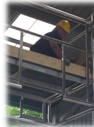
16. Fit toeboards in the correct position.
