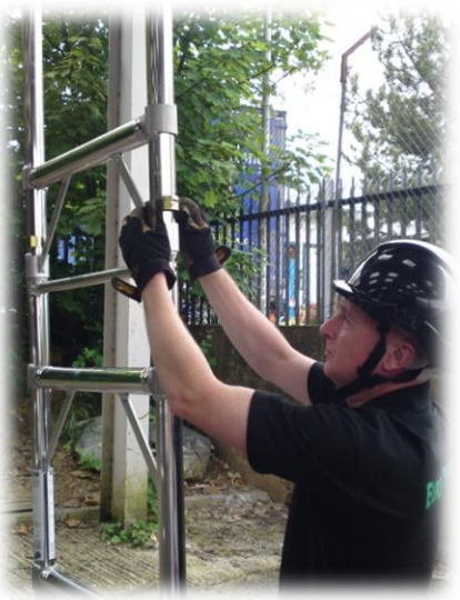
5. Engage Interlock Clips.
