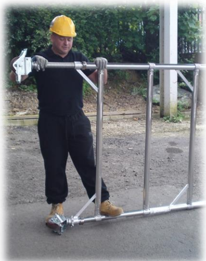
1. Insert 2 legs and castors into each frame.
