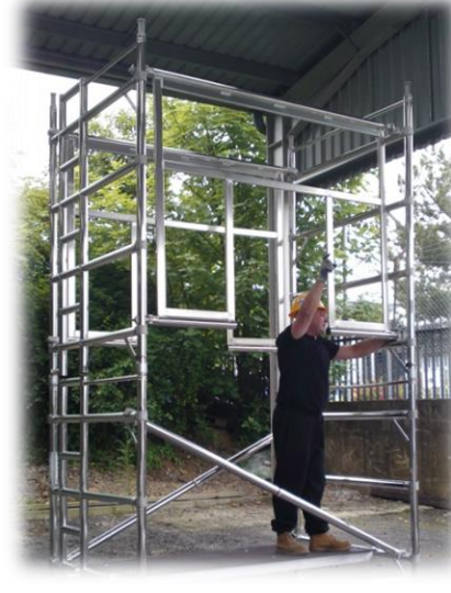
7. Standing on the platform, with the green label facing you, position the 1 st pair of AGR frames to the vertical members above the rungs in the required position as shown.
