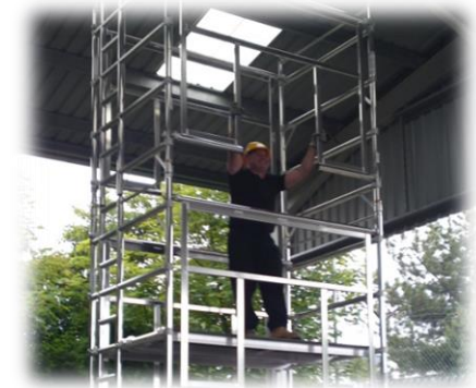
12. Safely pass up the next set of AGR frames as shown.
