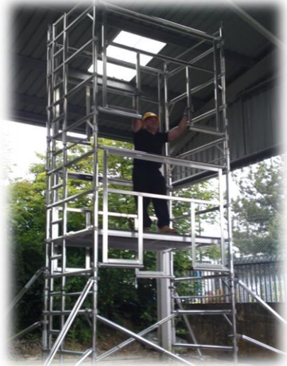
13. With the green label facing you, position the AGR frames to the vertical members, above the rungs in the required position as shown.
