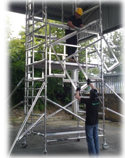
12. Safely pass up the next set of AGR frames as shown.
